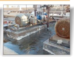
This high pressure acid pump containment area and its pump bases, located at a western U.S. geothermal energy plant, were crumbling and falling apart.
