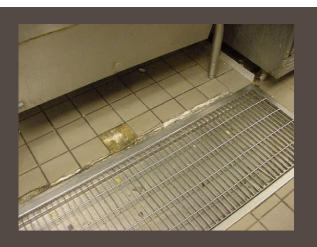
Portions of tiles where grout had failed were chipped away.
