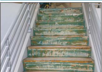
This indoor atrium staircase at a prestigious eastern U.S. university was falling into disrepair. The old vinyl tiles were detaching from the substrate causing an eyesore as well as safety concerns for students and faculty alike.
