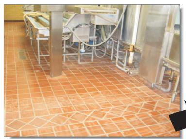
This tile floor located inside a New Jersey hospital's dish washing area had begun to deteriorate. Grout was wearing away, missing or had become porous allowing leaks from spilled water into the floor below.
