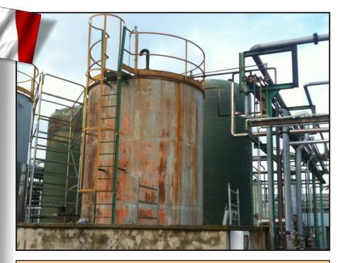
The chemical company needed to protect this tank which contains sulfuric acid (10%). Since grit blasting was not an option, mechanical wire brushing was employed. Three coats of ENESEAL CR were applied by roller (7 units). The client was delighted with the results.
