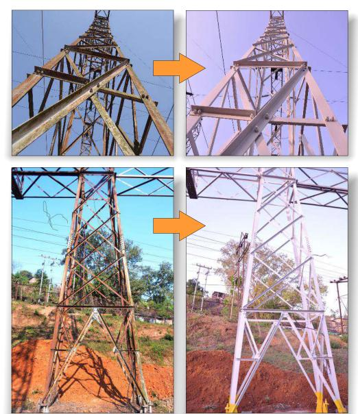
Built in the 1960's, these steel electrical towers were severely corroding because of the very humid and rainy weather in this region of India. The power company was looking for a cost effective solution to this on-going problem.
