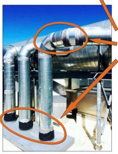
An area where these roof top air circulation pipes converge to enter a university building was vulnerable to leaks from rainwater. When this area leaked, water would drip down to laboratories below filled with expensive equipment.
