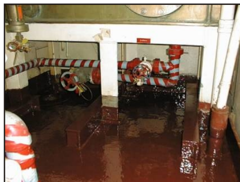
First coat of CeramAlloy Grey color followed by a second coat of CeramAlloy AFFF Red
