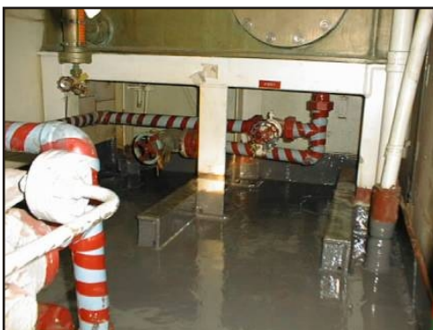
First coat of CeramAlloy Grey color followed by a second coat of CeramAlloy AFFF Red
