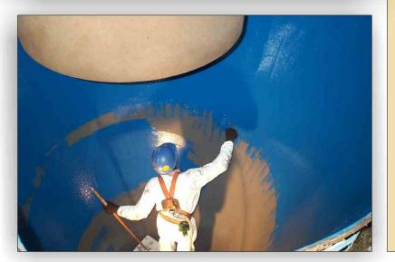
This large paper mill located in South Carolina wanted to repair and protect their wood chip cyclone separator. The engineers at the mill turned to their local ENECON distributor, ENECON South East, headed by Tripp Waynick.
