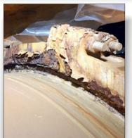
The coupling joints of these 48 inch diameter pipes were leaking. The pipes carry wastewater to clarifier tanks at the 5th largest wastewater treatment plant in the U.S. There are 12 of these pipes and they each have 3 couplings (36 total).
