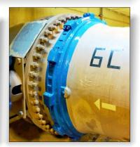
coupling area, followed by a final top-coat of CeramAlloy CL+AC (Blue) to completely seal and encase the couplings.
