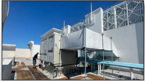
This rooftop air handler unit is located on the roof of 19 story building on the coast of western Florida. After years in service and exposure to an extreme salt air environment the unit was suffering from significant corrosion damage.
