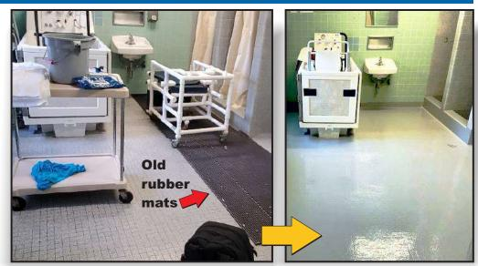
A hospital in eastern Pennsylvania was having a problem in a first floor bathroom that was leaking down into the basement below.
