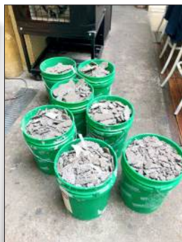
All the loose flooring material is removed
