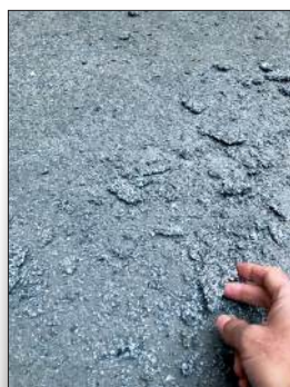
All the loose flooring material is removed
