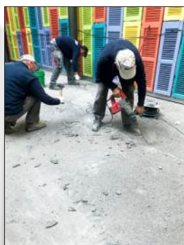
All the loose flooring material is removed
