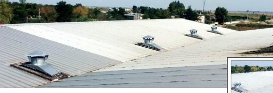
A shoe factory in Romania had a 45,000+ square foot metal roof that was leaking. Water was seeping through common problem areas near gutters as well as ventilation equipment protrusions.
