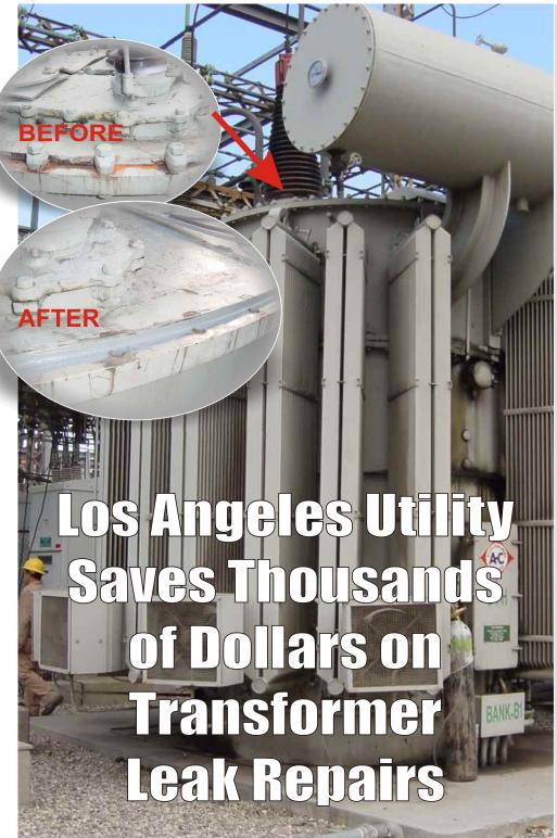
The top flange of this large transformer at a local Southern California electrical utility substation was leaking oil. The nitrogen blanket that normally covers the transformer oil rarely requires re-charging. However, due to the steady leaks, the utility had to hook up nitrogen cylinders to the transformer in order to maintain the nitrogen blanket over the oil.
