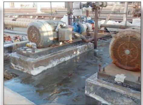
This high pressure acid pump containment area and its pump bases, located at a western U.S. geothermal energy plant, were crumbling and falling apart. These pumps are pumping 3% hydrochloric acid.
