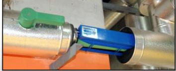
A local dealer for ENECON Italia in Malta, recently completed a long-term test with ENEFLOW at a major international hotel chain. ENEFLOW was installed on multiple water lines that were experiencing significant mineral scale problems.
