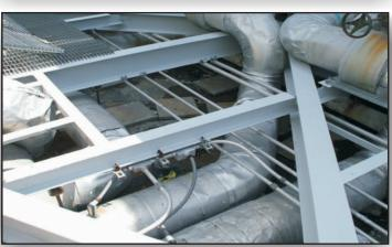
At this major pharmaceutical plant located in Pennsylvania, these 5 cooling towers sit atop I-beam supported grated platforms. These I-beams had been suffering for years from corrosion caused by atmospheric pollution mixing with the water splashing from the large cooling towers. The tight spacing of the grated metal supports also trap moisture and accelerate the corrosion problems.
