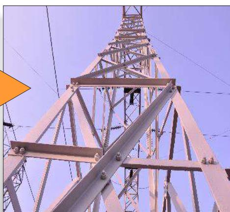
Built in the 1960's, these steel electrical towers were severely corroding because of the very humid and rainy weather in this region of India. The power company was looking for a cost effective solution to this on-going problem.
