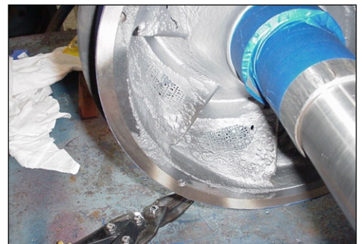
Reinforcing 'mesh' and DurAlloy applied over holes
