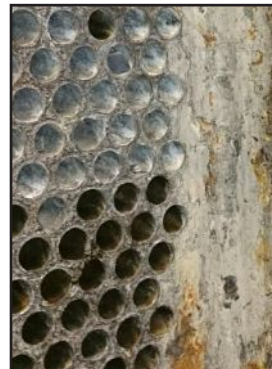
After grit blasting, METALCLAD CeramAlloy CP+AC was used to rebuild
