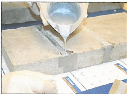
Filling horizontal cracks in concrete.
