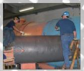
METALCLAD® DuraWrap® can be applied to the interior and / or exterior of piping and equipment to both seal and strengthen these components. When applied to the interior walls of underground or otherwise inaccessible piping, METALCLAD® DuraWrap® can effectively repair and restore piping integrity without expensive excavation and
