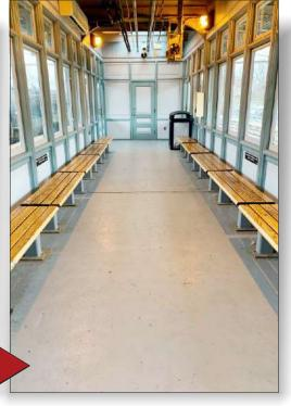
The above newsletter (CH-067) highlighted the repair and protection of a northeastern US commuter train waiting room floor completed 8 years ago. The surface of the floor was prepped and CHEMCLAD P4C was used as a primer. Two coats of CHEMCLAD GP were then applied with an aluminum oxide broadcast for slip-resistance properties.
