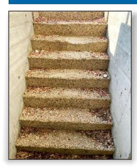
A western U.S. university had an outdoor staircase leading to a basement mechanical room that had fallen into disrepair. A previous attempt to repair the stairs had been made using an epoxy with an overlay of pea gravel. That repair eventually failed and the local ENECON Distributor was contacted and asked to help find a solution to this problem.
