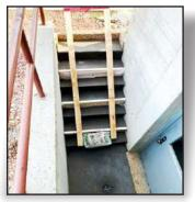
approximately 500 pounds of locally sourced sand was used to rebuild the staircase. The steps were given a proper pitch for water runoff.
