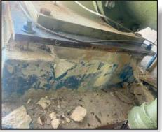
This concrete base supports a 350 hp, highservice vertical pump at a Florida water treatment facility. This type of pump has a total load of over 12,000 lbs. The municipality required a product with a high compressive strength and short downtime to complete this repair. The maintenance engineers at this facility had tried conventional repairs to similar bases and failed.
