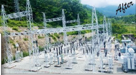
The power station's engineers needed a cost effective and reliable corrosion solution. They turned to the local ENECON distributor for help. The substation gantries were manually prepared then coated with ENESEAL CR. In all, approximately 1,900 square meters were protected at both substations.
