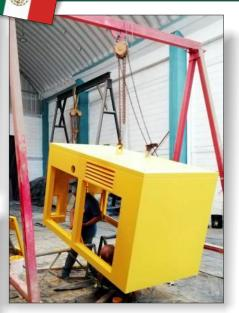
A local water authority in Mexico that supplies drinking water to the communities in the surrounding area had three water pumps that needed maintenance. To prevent further atmospheric corrosion damage to the pump's metal exterior casing, maintenance engineers asked the local ENECON Distributor to provide a solution.
