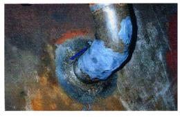
The area to be repaired is first thoroughly roughened using a grinder and rotary file. Then, using stainless steel mesh to bridge the actual holes, mixed METALCLAD SpeedAlloy is applied over these areas.
