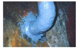
METALCLAD DurAlloy is then applied over the entire area, followed by Reinforcement Tape to "spiral wrap" the entire repair and more DurAlloy to completely cover the repaired area.
