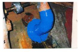
The application is finished off with METALCLAD CeramAlloy CL+ to encapsulate the DurAlloy and to protect any "bare metal" areas exposed during the surface preparation process.
