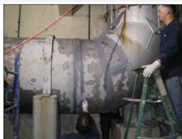
After grit blasting, leaks repaired with DurAlloy.
