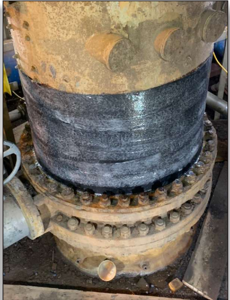
DuraWrap completes the repair.
