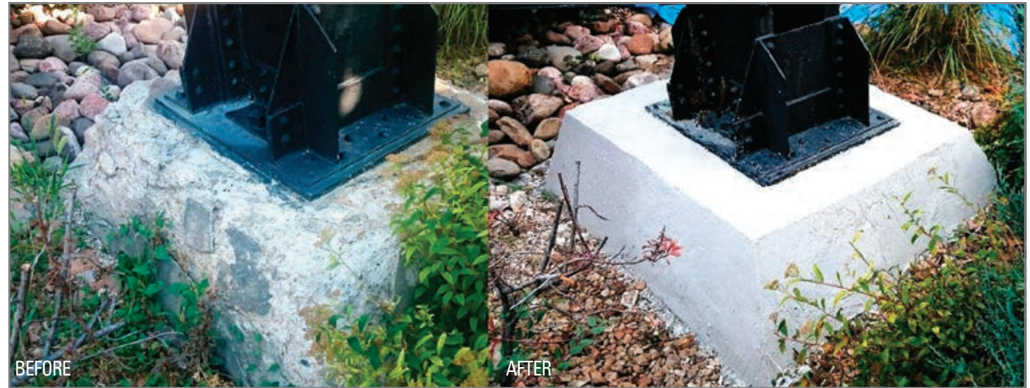
The applicability of concretelike polymer-based materials is widespread and can be beneficial when setting, securing or repairing areas around handrails, metal stair noses and footers.
