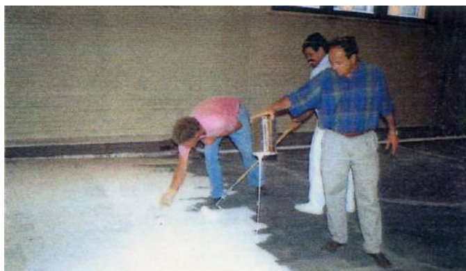
3. The application of CHEMCLAD P4C primer for concrete.
