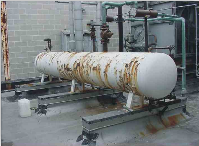
Badly rusted pressure tank and support legs. Project called for grit blasting tank and supports, then treating with CHEMCLAD SC (2 coats).
