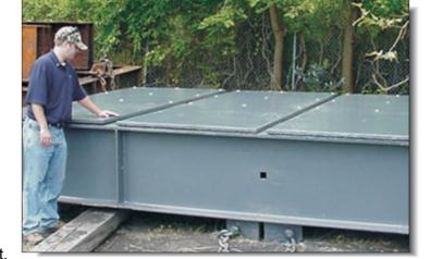
This 10 ton pier fender, used as a buffer between concrete pier pilings and boat hulls, was over 10 years old and suffering from severe erosion and corrosion due to constant exposure to salt water and tidal changes.
