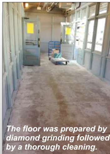
CHEMCLAD P4C was used to prime and seal the concrete surface.
