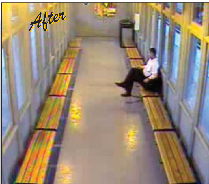
CHEMCLAD GP was applied and aluminum oxide was broadcast on the floor and back-rolled in to provide slip-resistance.
