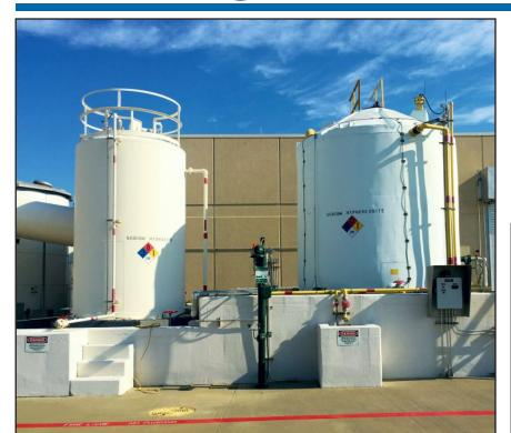
CHEMCLAD SC Protects Concrete Containment Area From Exposure To Sodium Hydroxide
