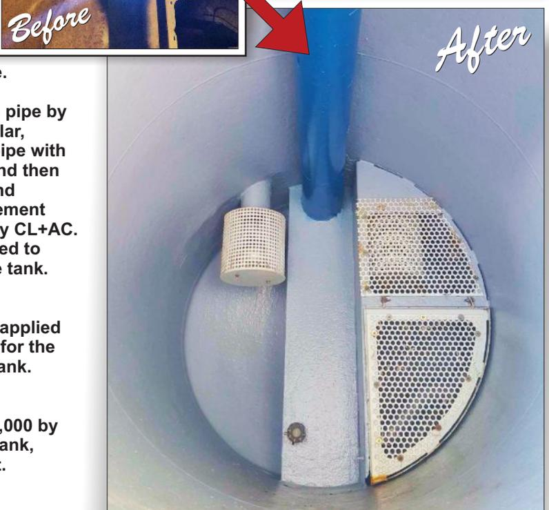
A Florida municipality which uses ENECON products for many of their repair and preventative maintenance needs had a problem that needed to be solved. A 1,500 gallon steel vacuum truck tank's interior was completely rusted and in desperate need of a solution.
