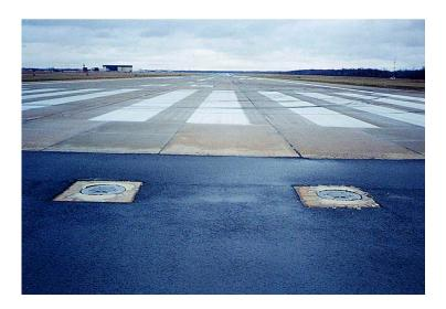
These concrete pads for these airport runway lights were badly deteriorated from service conditions subjecting them to freeze/thaw cycles, deicing salts and mechanical damage.
