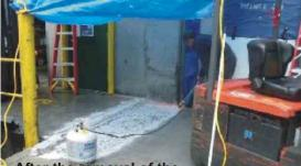
After the removal of the previous repair, the damaged area was abraded, cleaned and dried with a propane torch.
