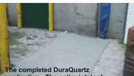
application. The entire job took about 4 hours with 2 men. The area was put back into service just 12 hours after finishing the repair. Years of settling and heavy forklift traffic had created approximately 4" of damage between concrete slabs on the cold storage loading dock at this Seattlebased seafood processor.
