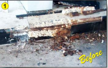
A very popular chain of ENECON Field Pennsylvania gas stations & convenience stores was experiencing severe corrosion and erosion on their gas pump island curbs. It was a potential hazard to customers and employees in addition to being very unsightly.
