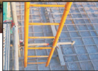
SuperBond Sprayed Over Existing Concrete & Reinforcing Bar.
