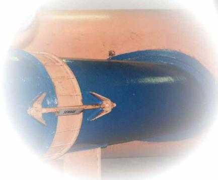
The ENECON North East Engineering Team was given a daunting challenge: to salvage this main pumping station's discharge pipes which were developing leaks due to the aggressive effluent as well as the age of the pipes, themselves.
