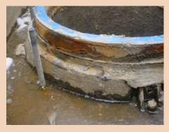
These two concrete manhole covers over the power station's main cooling water intake lines were in very poor condition. It was impossible to keep these sealed. So much water was leaking through the covers that sump pumps had to be used constantly in order to keep the pit from filling up with water.
