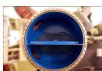
These heat exchangers at a Silicon Valley data center circulate reclaimed water, which contributes to accelerated erosion and corrosion.
