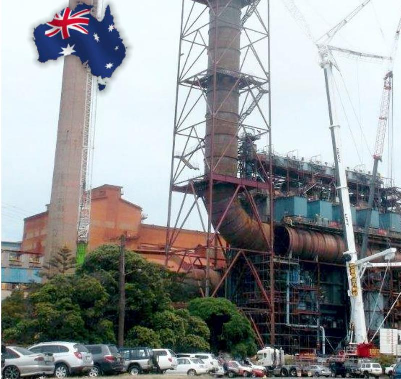
Waste gas from the steel making process is treated at this Australian waste gas cleaning plant. A new steel exhaust stack was being installed and the plant's engineers wanted to protect the 90 degree bend in the stack (also known as the "lobster back") from the extremely corrosive environment.
