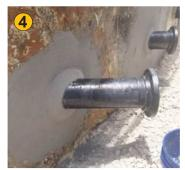
The repaired pipes and tank wall.
