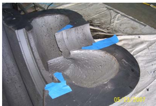
Figure 3-3 Interior after Sandblasting
