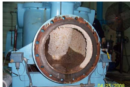
Figure 5-4 Interior Suction Side
