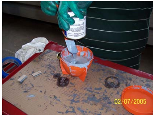
Figure 8-7 Mixing of Belzona
