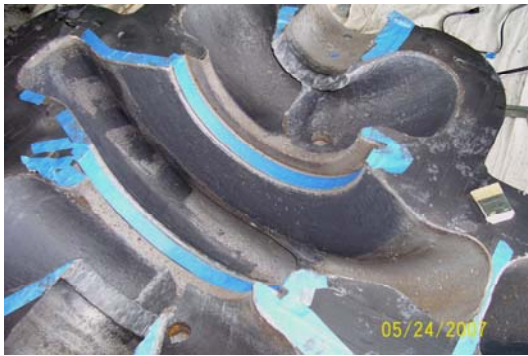
Figure 3-4 Interior after Metal Filler
