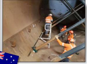
Upon inspection it was discovered that the exhaust duct of this Australian waste gas cleaning plant was suffering from significant corrosion. Originally 8mm thick, accelerated corrosion had resulted in a significant reduction in thickness and several holes throughout the duct.
