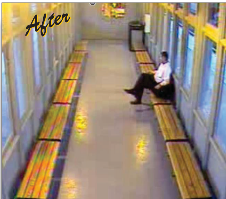
CHEMCLAD SC was applied and aluminum oxide was broadcast on the floor and back-rolled in to provide slip-resistance.
